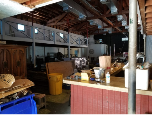
Post 168, Downtown Key West—Recovering from Irma Damage
